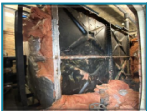
Before and after - Trove Court water tank replacements
